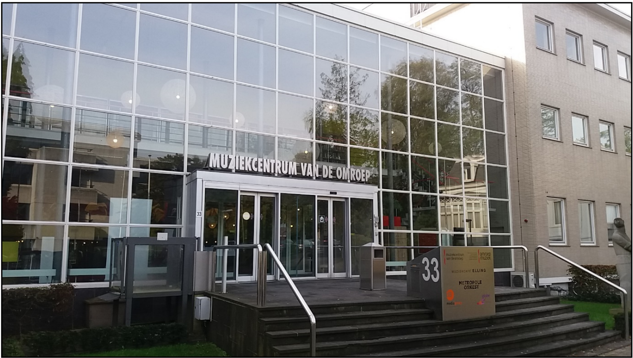
Entrance of the music center in Hilversum
